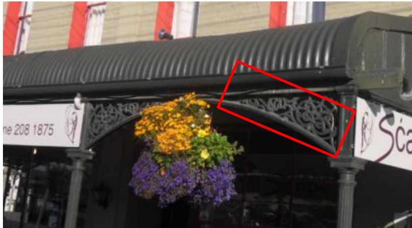
Figure 4 Haunches have been removed
