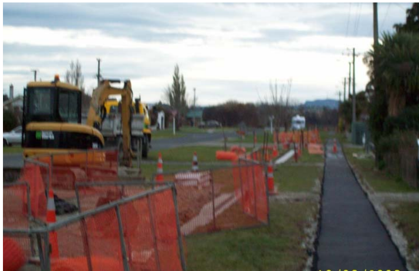
Asphalt footpath reconstruction underway in Nelson Street
