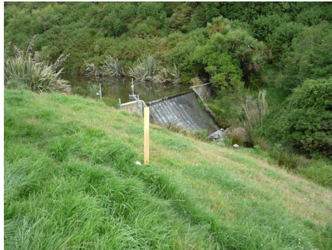
Photo of Pleura Dam
