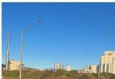
Figure 2: Current view from Northeast side of Plant
