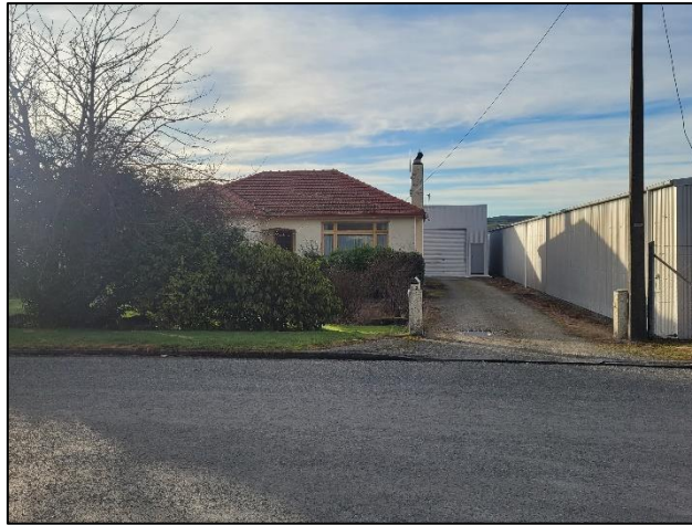
Figure 5: 12 Rata Street, as viewed from Rata Street (photo – taken in July 2023)
