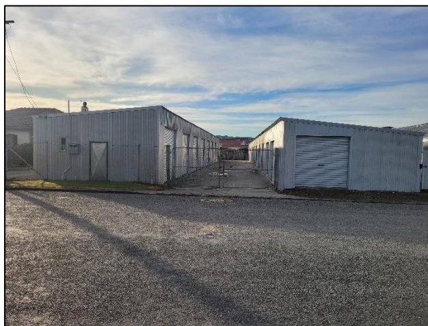
Figure 6: 14 Rata Street, as viewed from Rata Street (photo – taken in July 2023)
