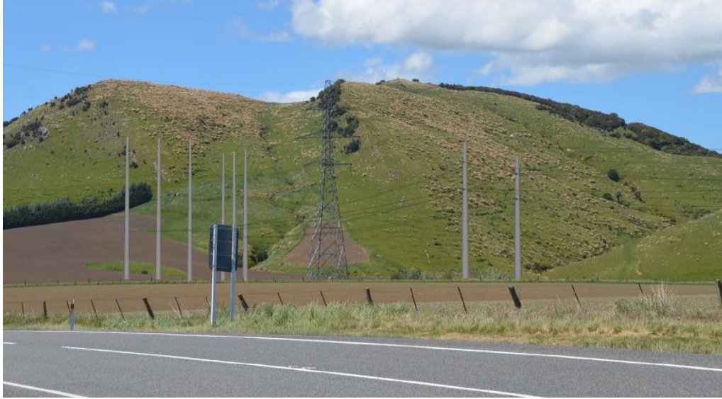
Figure 4: View of the Consented Eight-Pole Transmission Connection at Tower 139 of the NMA-TMH
