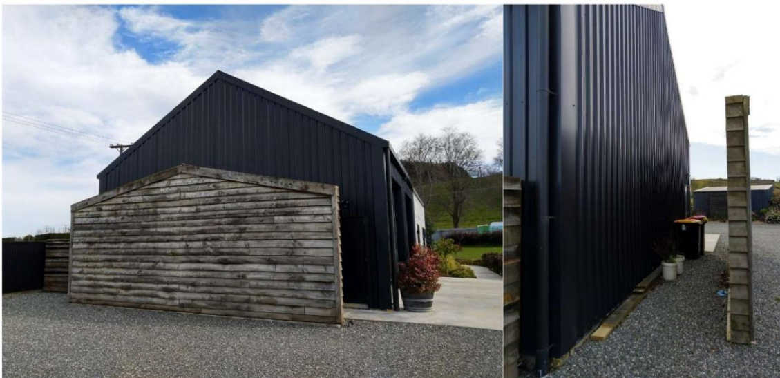
Figure 2: View of dwelling and free standing wall fence
