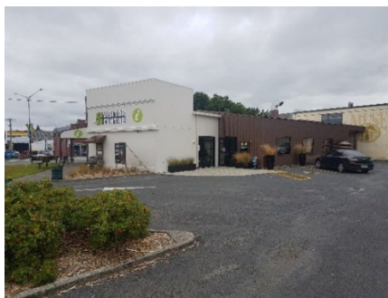
Functional entrance to relocated Gore Visitor Centre
