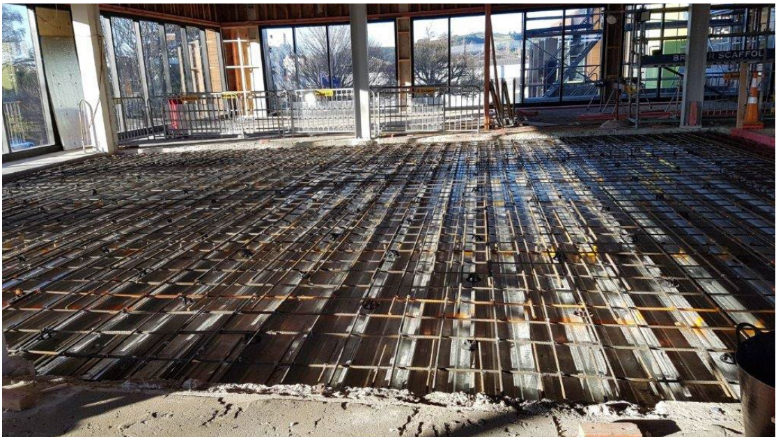
Upper-level floor prior to concreting on 6 July
