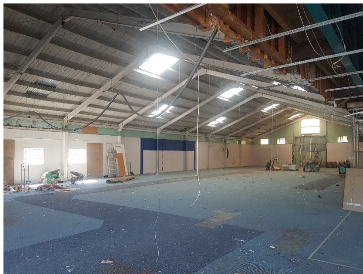
Cleared interior at 7 Norfolk Street
