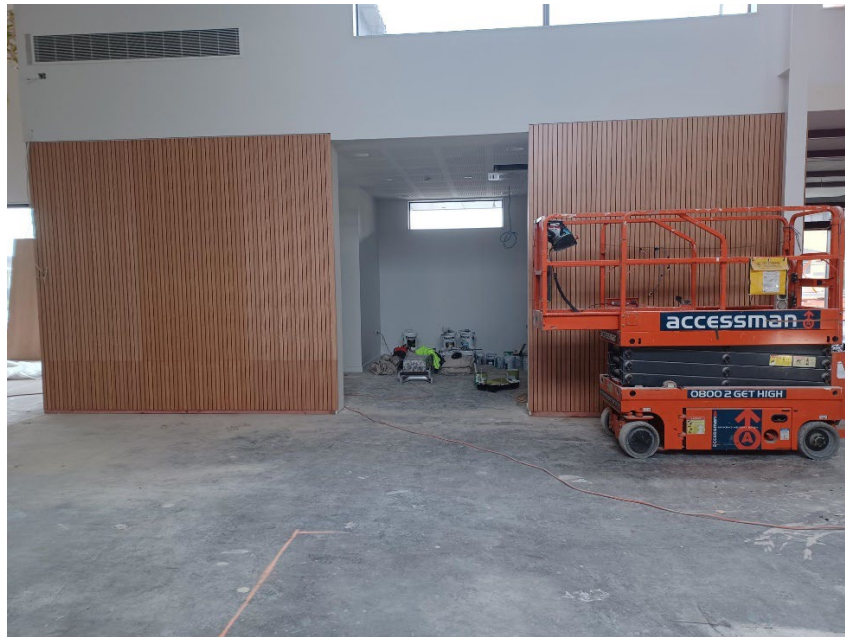
Entrance to the teen area, ground floor
