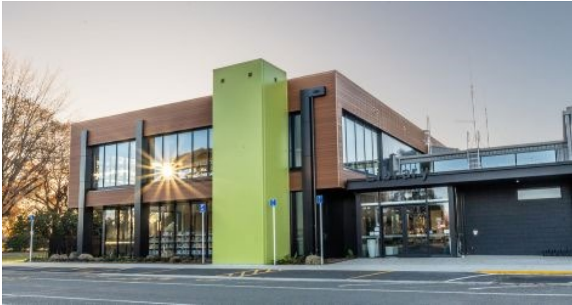
Some recent photographs of the new Gore Library building
