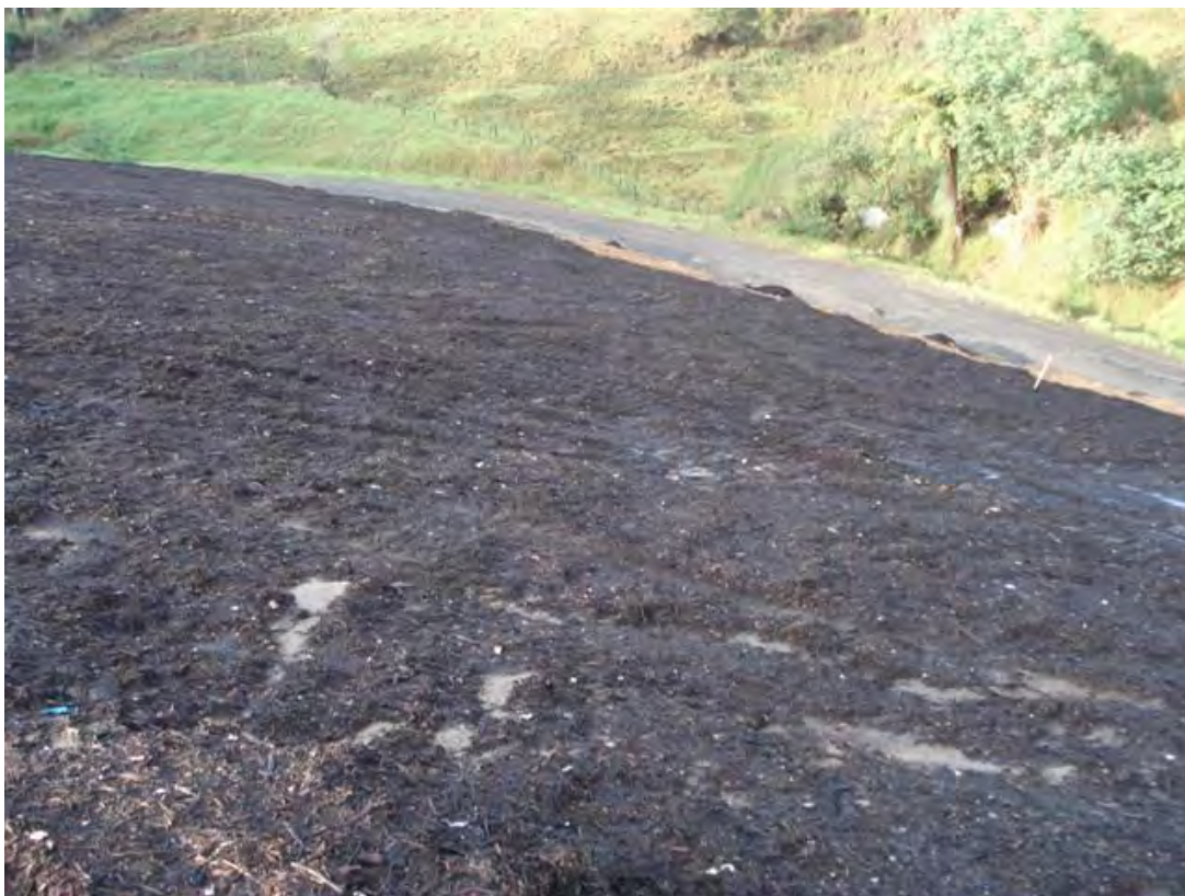
Photo 2: Close up of mulch following intense rainfall. Some localised patches where mulch had moved but overall, the site was in excellent condition considering the rainfall and the underlying capping soil was undamaged.
