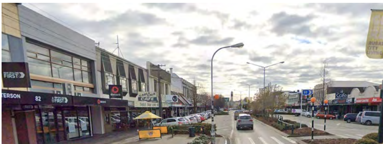
FIGURE 15 – LOOKING NORTH FROM THE INTERSECTION OF MERSEY AND MAIN STREET – TOWARDS THE COMMERCIAL CORE
